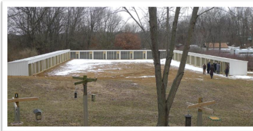
The 36 unit mew complex as seen from the IRC conference room.
